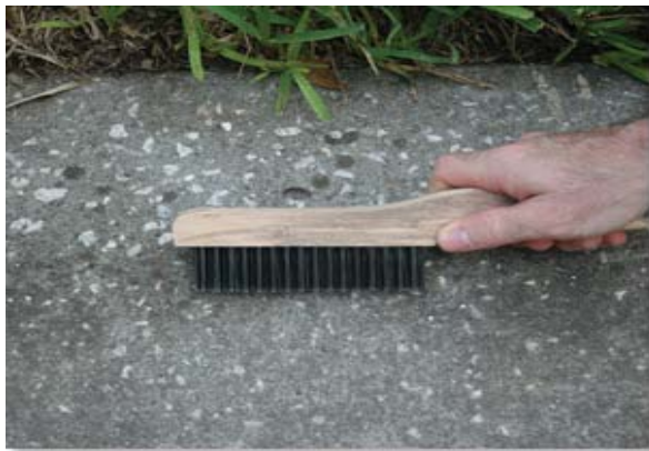
Optimum temperature is 40° F minimum to 90° Surface should be clean and dry
