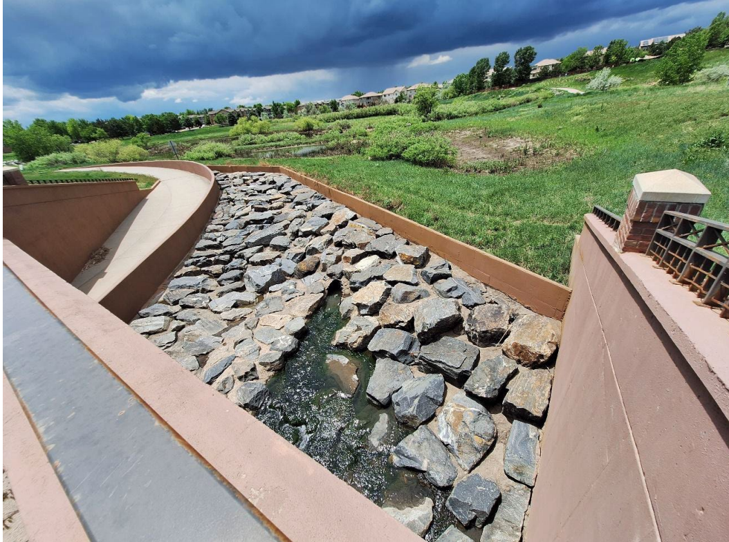
Spillway Crestwall (SC-1), Grouted Boulders, and Floodwall (Map ID: J for Crestwall; Floodwall and Concrete Trail Owned by Others)
