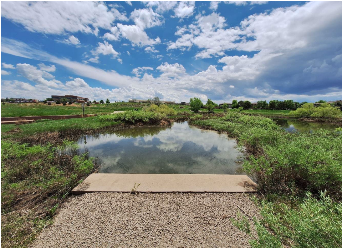
Outlet Structures No. 1, Micropool, and Wetland Bench (Map IDs: H, F, E)
