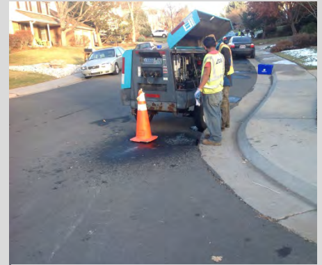
Investigating a hydraulic fluid spill from a residential generator, requiring cleanup and abatement
