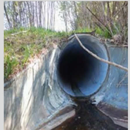
A rehabilitated corrugated metal pipe outfall
