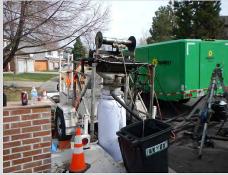
The Cured-in-Place (CIPP) pipe technology
