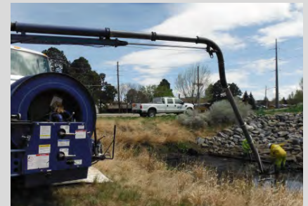
Cleaning outfalls & inlets with the Vactor® truck
