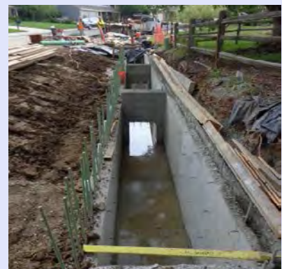
Additional storm sewer pipe to move water from the streets to the system
