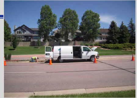
Camera Van televising storm sewer pipe system
