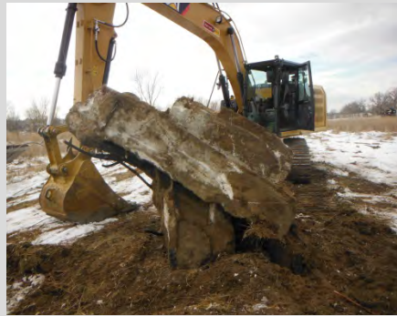
Removing an illegal bridge obstruction in the Piney Creek floodplain to resolve a permit violation; a designed pedestrian bridge will be built as part of a CIP project.
