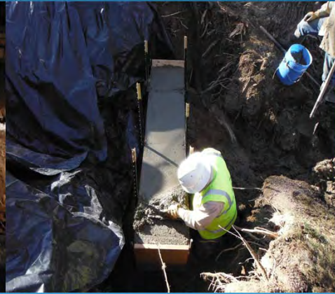
Cutoff Wall Construction
