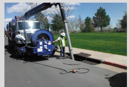
Cleaning outfalls & inlets with the Vactor® truck
