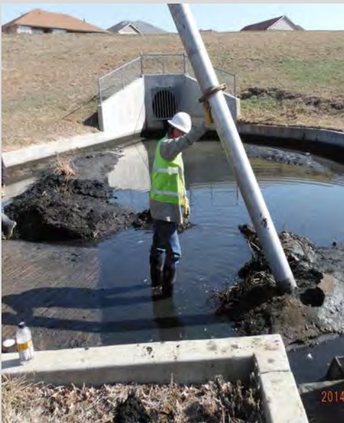
Cleaning sediment collected in detention pond forebay
