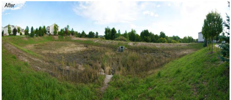
Southcreek Pond A showing an anoxic boggy bottom and sparse vegetation in March 2013, as compared to the newly constructed retrofitted pond in September
