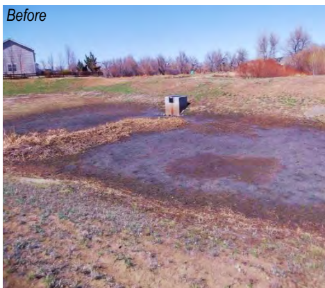
Southcreek Pond A showing an anoxic boggy bottom and sparse vegetation in March 2013, as compared to the newly constructed retrofitted pond in September
