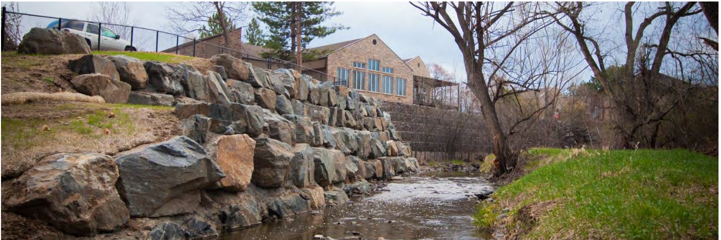
This grouted boulder bank protection provides stability during high flow events in Little Dry Creek for the Southgate Water & Sanitation District offices in Centennial
