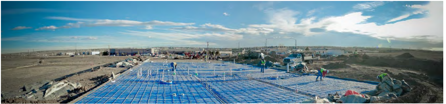
The SEMSWA building under construction adjacent to Regional Pond D-2.
