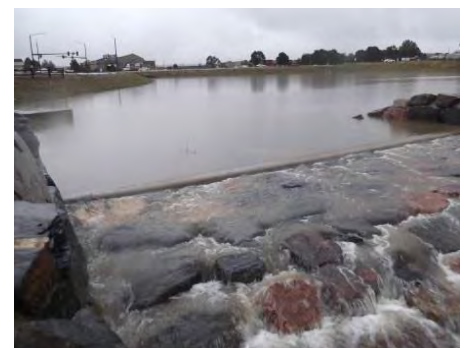
Regional Ponds in the Cottonwood Creek, Dove Creek, and Windmill Creek basins detain storm flows and release at a slow rate to keep the runoff peaks from damaging structures
