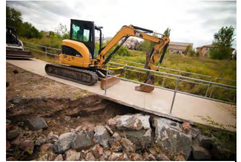
Emergency repair of Piney Creek eroded banks
