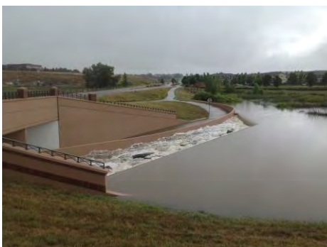
Regional Ponds in the Cottonwood Creek, Dove Creek, and Windmill Creek basins detain storm flows and release at a slow rate to keep the runoff peaks from damaging structures
