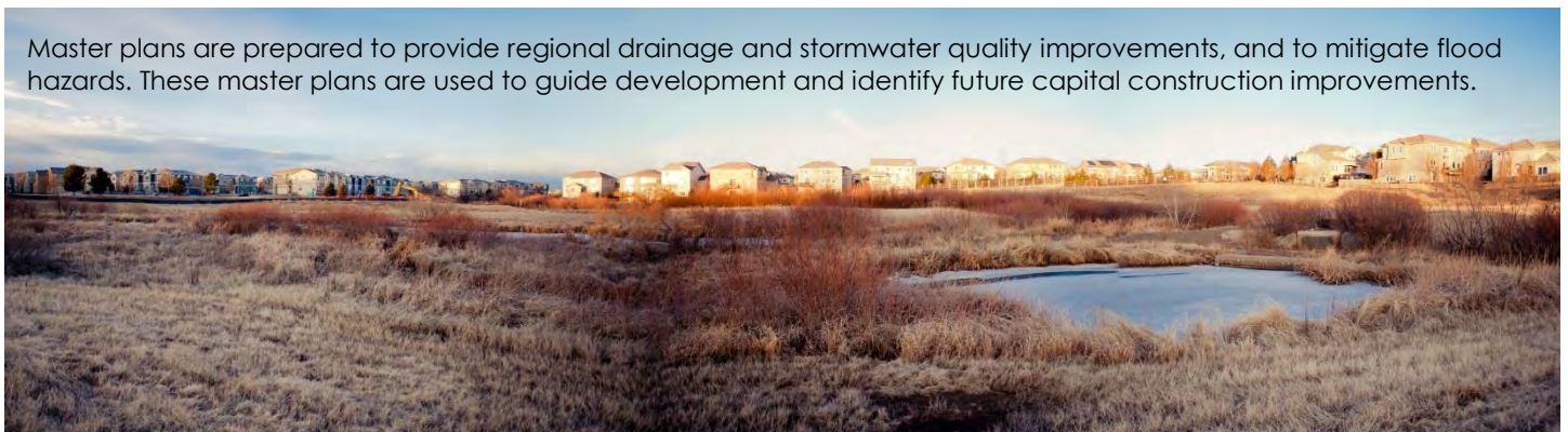
One of the regional pond facilities along Cottonwood Creek, a basin that has been master planned with larger, more effective ponds for flood control detention
