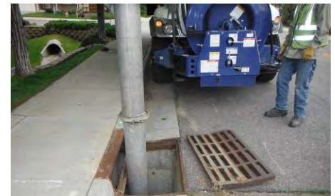
Cleaning inlets with the SEMSWA Vector® truck
