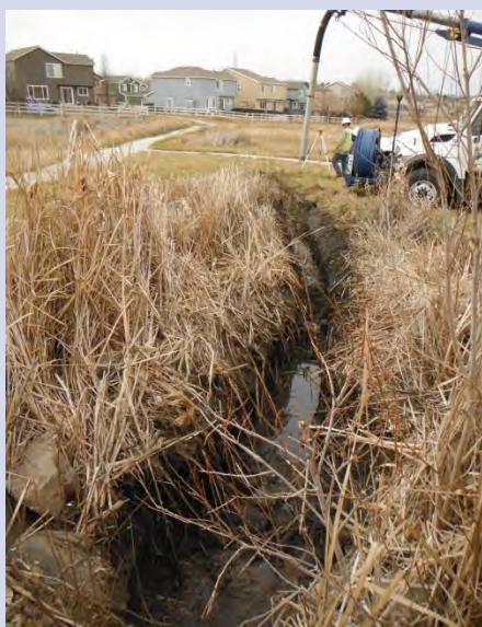
Cleaning sediment at the Kenyon Street outfall
