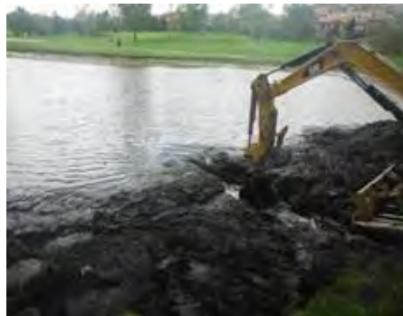
Maintenance crew releasing storm flows from pond
