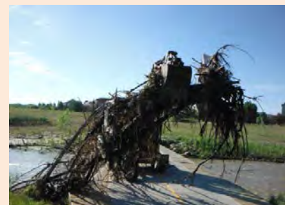
Forebays/channels require routine maintenance, including annual sediment & debris removal
