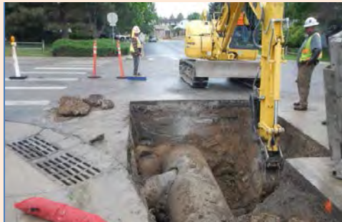
Undersized and deteriorating culvert crossings under Rosemary Way, carrying tributary flows to Willow Creek, required upsizing to safely convey storm event flows
