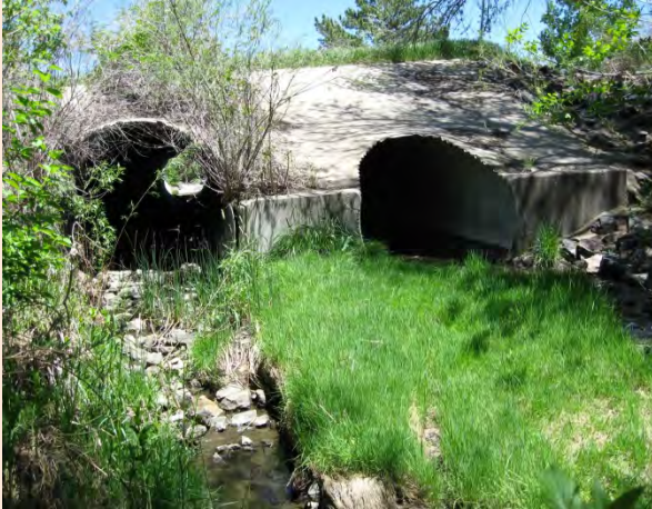
Undersized and deteriorating culvert crossings under Rosemary Way, carrying tributary flows to Willow Creek, required upsizing to safely convey storm event flows
