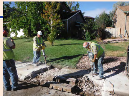
Prepping a street inlet for concrete repair work
