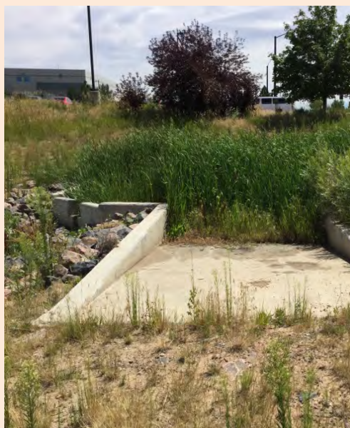
Vegetation can also impede detention basin function
