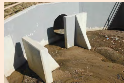
Forebays/channels require routine maintenance, including annual sediment & debris removal
