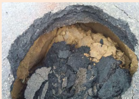
Sinkholes are associated with a void that develops in the vicinity of a storm pipe; in this instance, a pipe that takes storm flows off County Line Road at Chester Street
