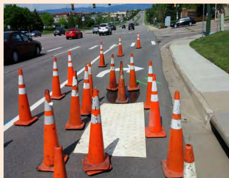
Sinkholes are associated with a void that develops in the vicinity of a storm pipe; in this instance, a pipe that takes storm flows off County Line Road at Chester Street
