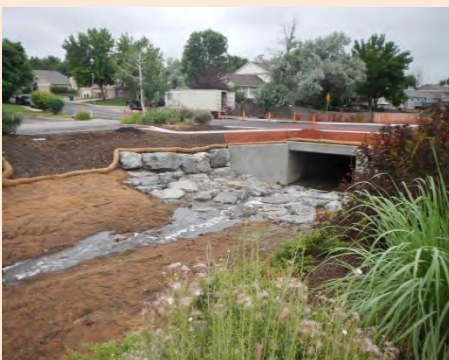
Completed South Rosemary Way Culvert Crossing
