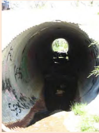
Undersized and deteriorating culvert crossings under Rosemary Way, carrying tributary flows to Willow Creek, required upsizing to safely convey storm event flows
