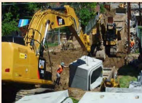
Contractors worked in back yards to install pipe
