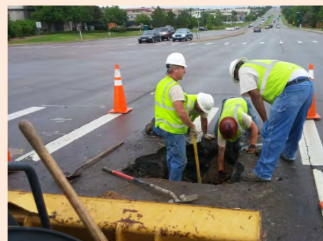
Sinkholes are associated with a void that develops in the vicinity of a storm pipe; in this instance, a pipe that takes storm flows off County Line Road at Chester Street
