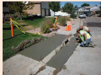
Putting final touches on concrete replacement
