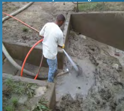
Vacuum Truck Dump Pit Cleaning
