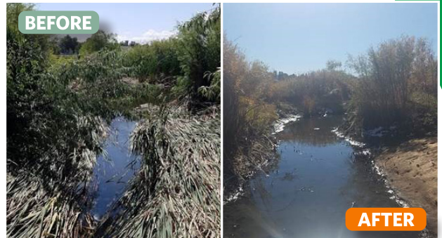
Example vegetation removal to improve flood flow conveyance in channels (above) and storage capacity in regional ponds (below)
