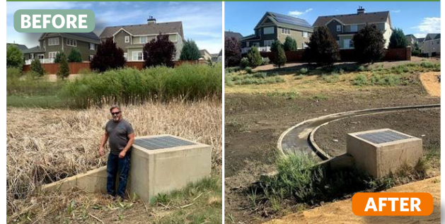
Example vegetation removal to improve flood flow conveyance in channels (above) and storage capacity in regional ponds (below)
