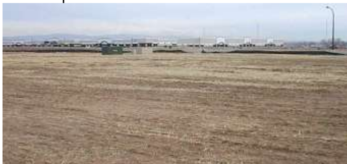
This site was issued a re-inspection fee when the GESC Manager scheduled an inspection prior to reaching the required vegetative cover as well as not maintaining the required sediment controls.
